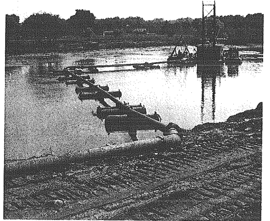
Monument with pontoons: The Pumping Derrick. (Photo: Robert Smithson.)
